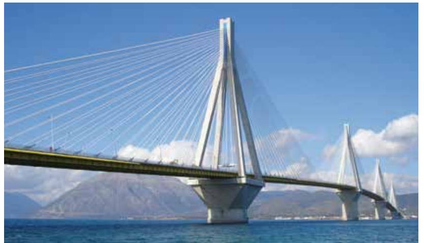
Harilaos Trikoupi Bridge, Greece
